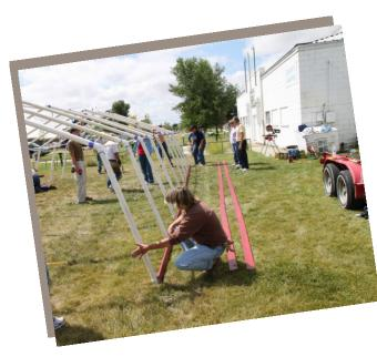
The 10 foot boards are on the outside and the 12 foot board is in the inside. With a brace splice the wood together. There are 3 sideboards per side. Place a side board on the ground at the end of the legs.
