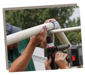
Add 18 inches of <sup>3</sup>/<sub>4</sub> inch PVC pipe to each side. Mark this pipe every 4 foot part and attach the tubular braces to the top of the structure using conduit clamps. Cut off
