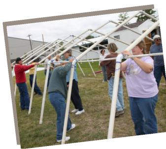
If you are not using the tubular braces for irrigating, you can attach the tubular brace directly to the 2 in. pipe using a 2-in. decking screws. If you will use the tubular brace for watering, you must use a <sup>3</sup>/<sub>4</sub>-in. one-hole or two-hole conduit clamp to attach the pipe.
