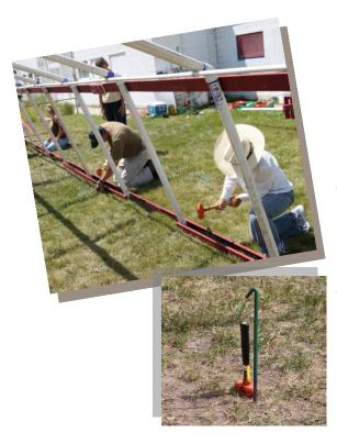
When boards are in place, drive two 24 inch. Rebar stakes bent in a "J" design over each board. This will help keep the hoop house anchored during high velocity windstorms. Repeat process on other side.
