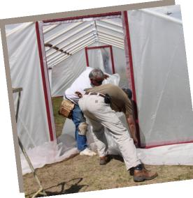
Cut the plastic out of the door frame and set aside until making the door. On the bottom of the hoop house cut all excess plastic to 1 foot out and remove the rest.
