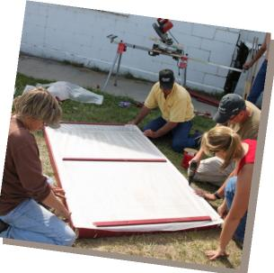
Attach two 3 inch hinges to the side of the door and hang the door in the door frame. On the inside of your hoop house door frame attach 1 inch x 4 inch boards. This will keep air from entering around your door.
