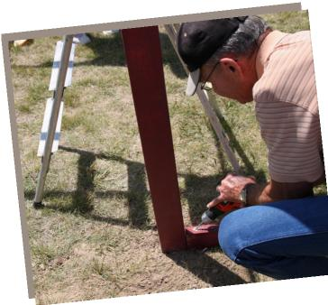
On the ground set a 2inch x 4 inch board from the door frame to the structure. Secure these boards by using 3 inch screws. This board gives support to the hoop house and the plastic will also be attached to it.
