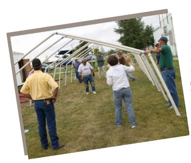
If the rebar stakes are perpendicular to the ground, it is very difficult to place the pipe on the spike. That is why stakes should be placed at a 30-degree angle. Place all 9 ribs on the stakes.
