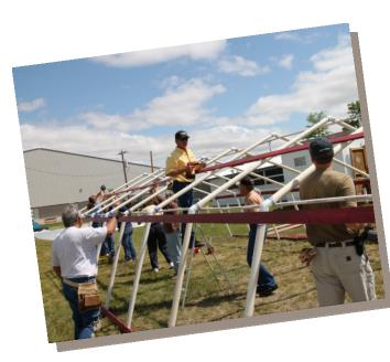
Place another sideboard half way in the middle of the rafters, the length of the building. Secure the bottom side board to a 2 inch plastic pipe.
