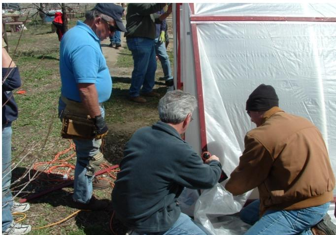
Stretch the plastic in both directions and use 1/2 inch thick by 1 1/2 inch wide by 8 foot painted wood strapping 'slats' and attach to the base board with the plastic sandwiched in between using 1inch zinc plated screws .. Repeat with the side board. When you have finished one side repeat it on the other. For the ends, stretch the plastic tight and attach the strapping to the 2 inch PVC pipe using 1inch zinc plated screws o one foot
